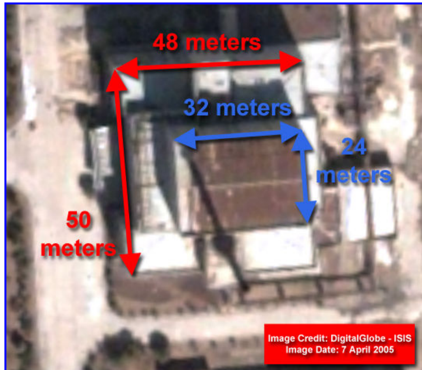
Figure 4. The five megawatt electric reactor building at Yongbyon, North Korea.
